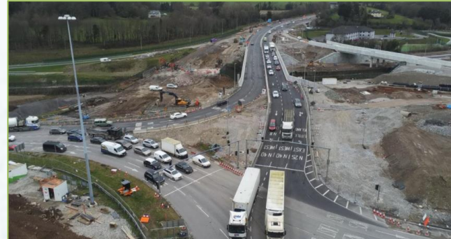
Dunkettle Interchange works
